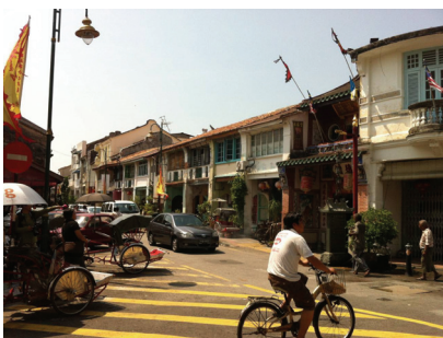
Fig 2. Location site of the 10 shophouses at Armenian Street
